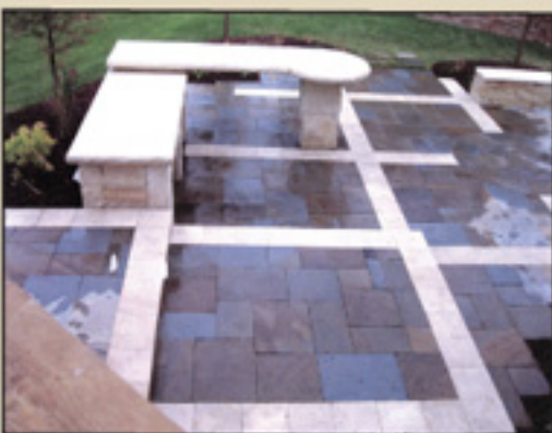
Geometric patio using Natural Cleft Bluestone - Random Ashlar pattern. Stonework by Urban Oasis, 913-660-4684.
