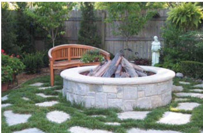
(Above) Fire Pit with Indiana Limestone cap, Colonial Gray building stone and Antique Gray flagstone stepping stones.
