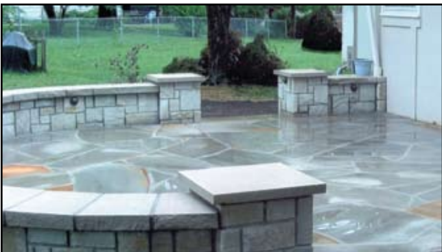
(Above) Misty Blue flagstone and Classic Gray veneer stone with Indiana Limestone cap. Photo/Stonework by Landscape, (816)985-2233
